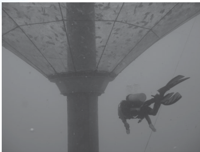
Each of four growout cages, located a half-mile offshore from the Big Island's Keahole Point and submerged 30 feet below the ocean surface in water 200 feet deep, hold up to an estimated 110,000 fish.
