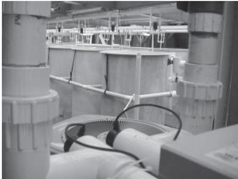
FIGURE 1. *Photograph of new replicated flame angelfish broodstock system showing several of the broodstock tanks in the background and heat pump and UV sterilizer in the foreground.*
