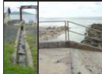
Effluent drain (Pohnpei, FSM)
