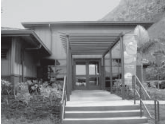
Entryway to the Information Technology and Training Facility
